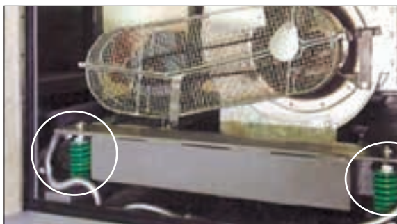
Blower in AHU on Open Spring Units
